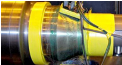
Turbine shaft dimensional restoration
