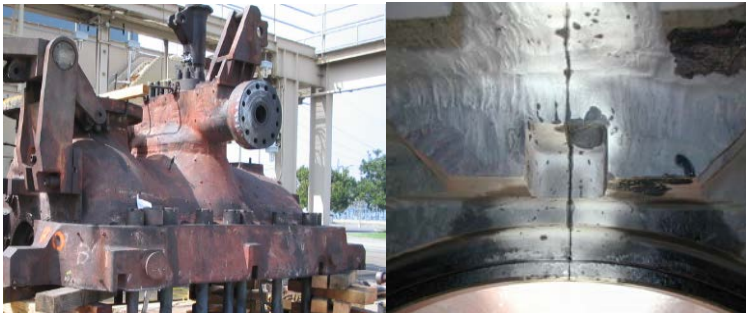
Steam Turbines cracks, steam cuts.....
