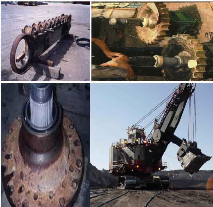
Dragline (Shovel) oversized bush housings and sprocket drives restored.
