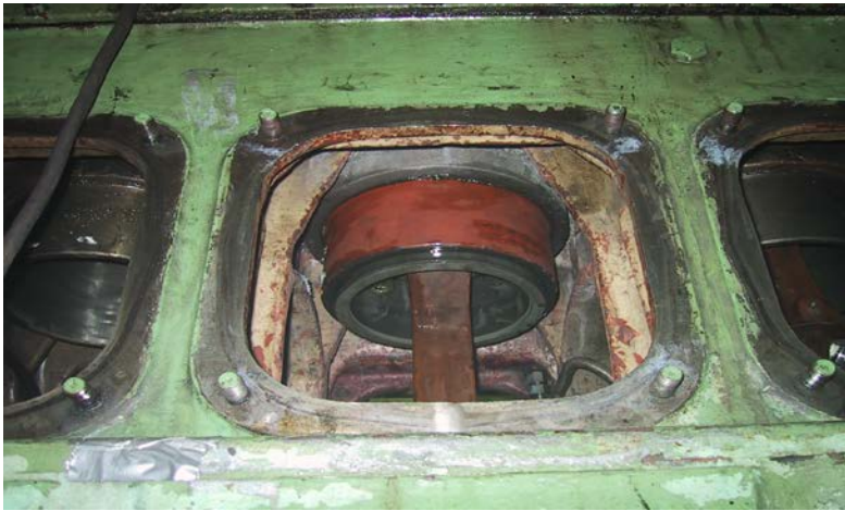
8 MW Marine Engine Block fully restored after cylinder area catastrophic failure.
