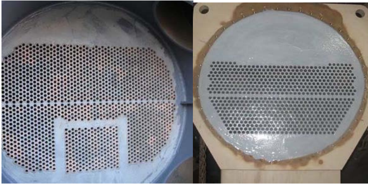
HX tube sheet and water box repair and special coatings to protect against bi-metallic corrosion
